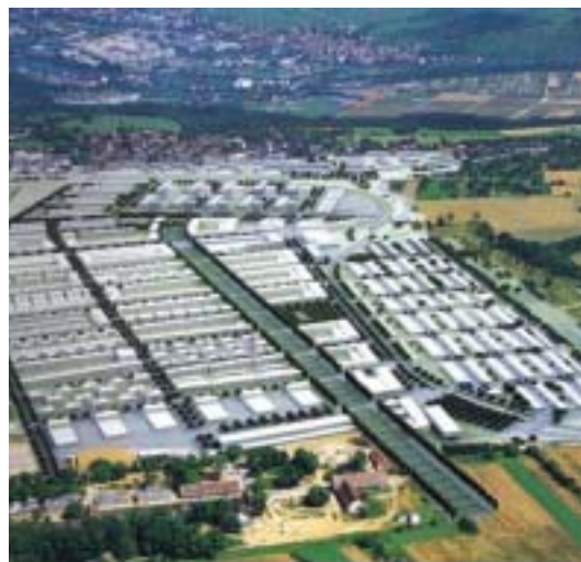
ABB. 29: OSTFILDERN SCHARNHAUSER PARK
